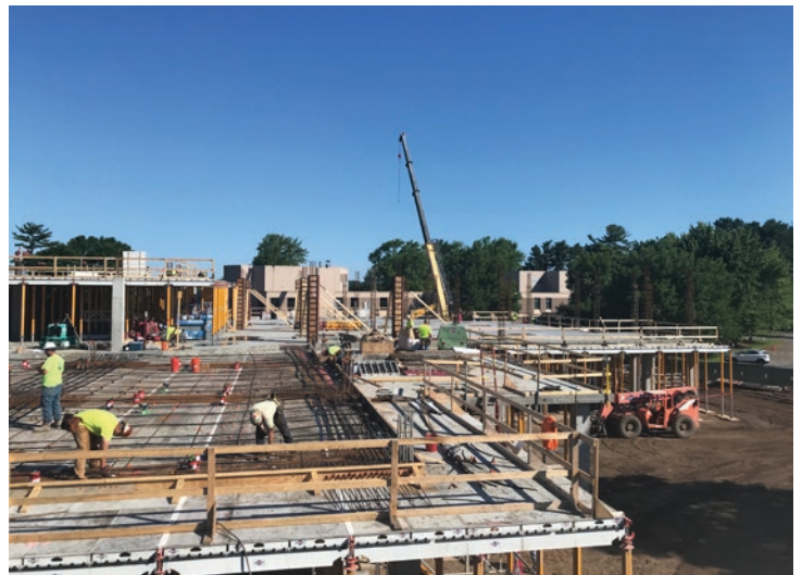
Youth Hospital Patio Fencing
